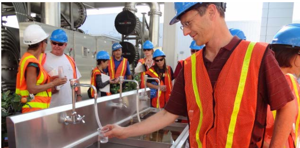
At locations like Orange County Water District (above) and West Basin Municipal Water District, indirect potable reuse plants are operating and visitors can taste the highly purified water.
