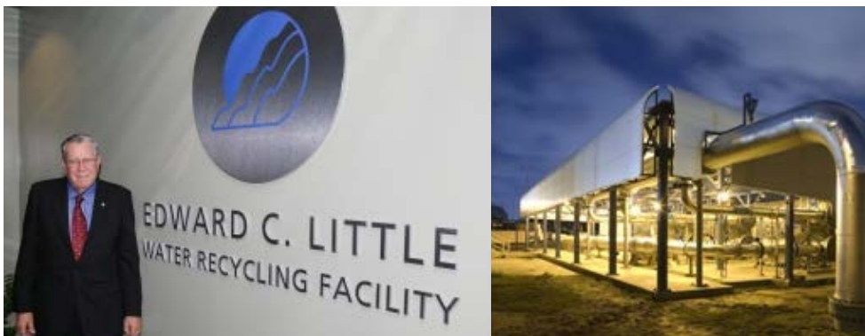
West Basin's Water Reliability 2020 program is designed to shift their future water supplies to more locally controlled and reliable sources of water. Their Edward C. Little Water Recycling Facility produces five different qualities of "designer" or custom-made recycled water that meet the unique needs of West Basin's municipal, commercial and industrial customers.
